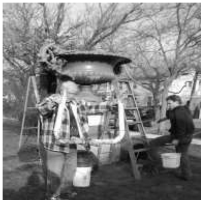
Removing a pipe from the urn for repair work
